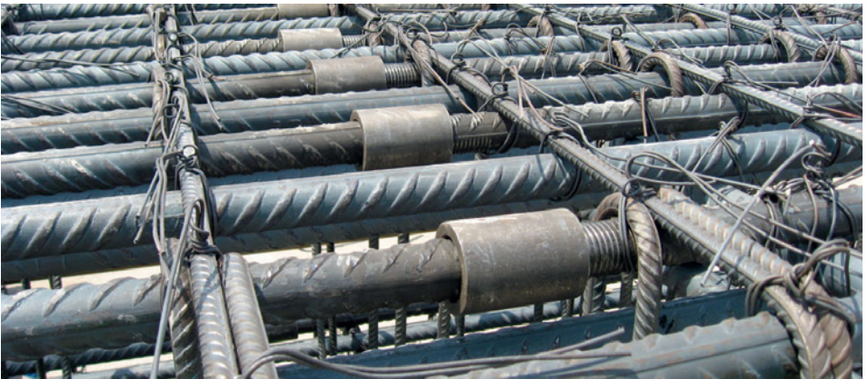
Figure 2. The use of rebar couplers can reduce rebar congestion as it eliminates the requirement to lap rebar.
